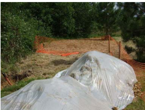
Exploratory dig site to locate damaged cable and repair it
